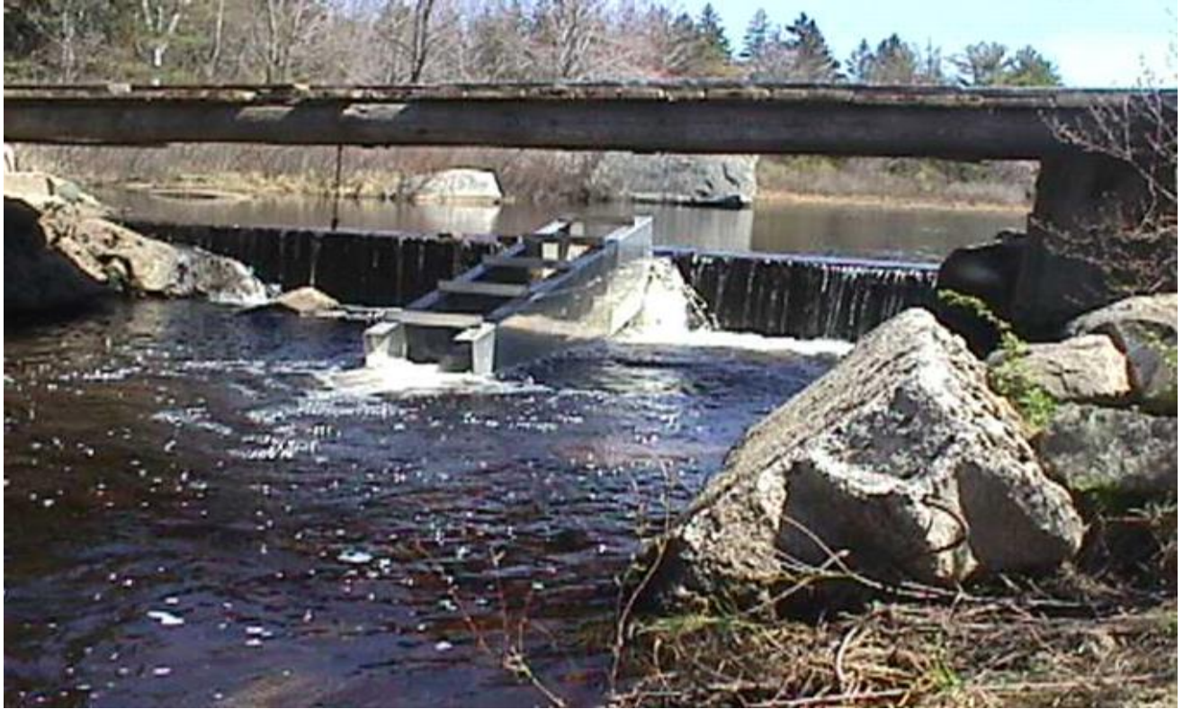
Old dam and fishway located at Wights Pond prior to installation of a nature-like fishway
