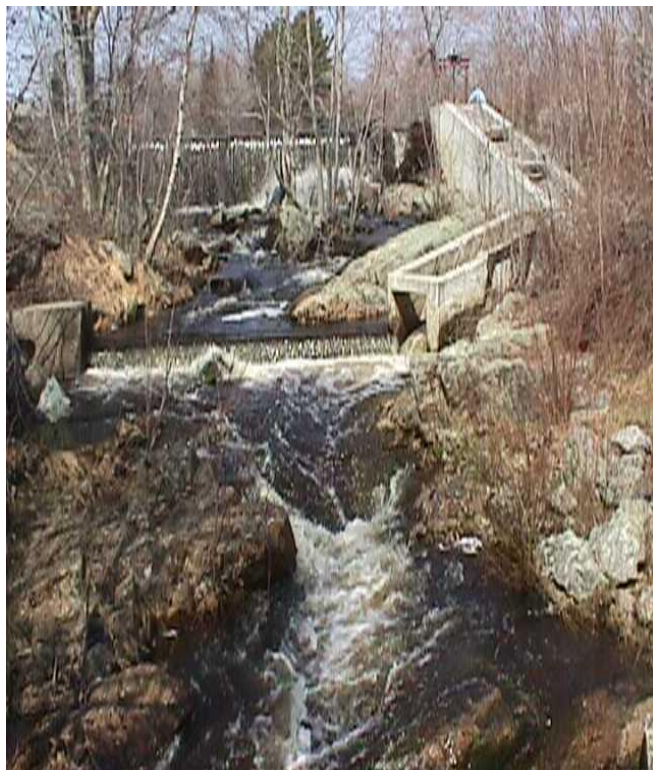
Fishway, fishing location, and trap deployed in the Gouldsboro alewife fishery.
