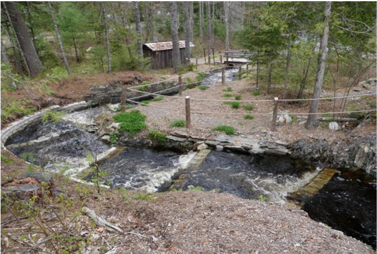
Lower fishway constructed below the dam
