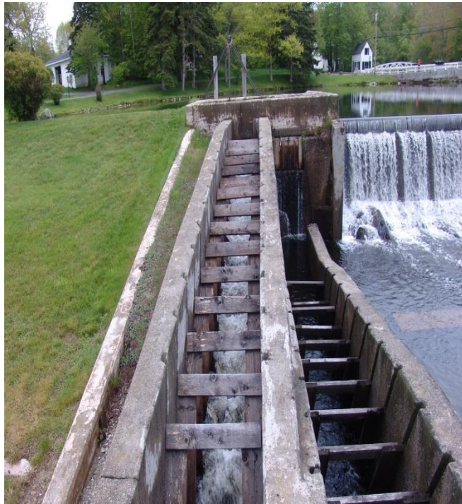
Tidal Denil fishway located in Somes Harbor and Somes Brook leading to Somes Pond.
