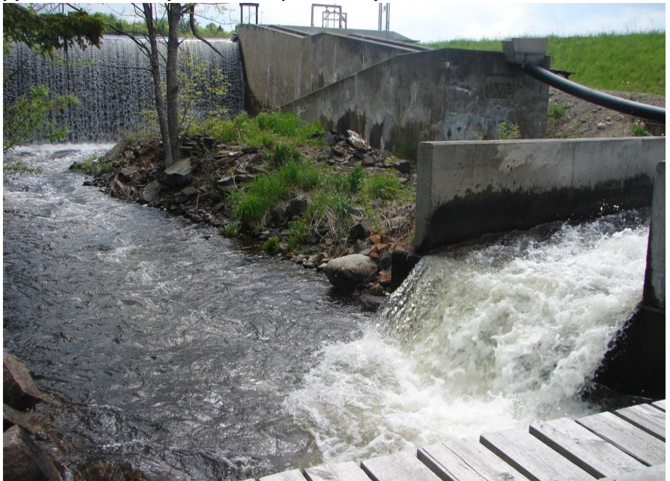
Dam and fishway under high flow conditions in 2006. Note harvest box and sluice pipe located at the corner pool of the fishway used to transport harvested fish into totes.
