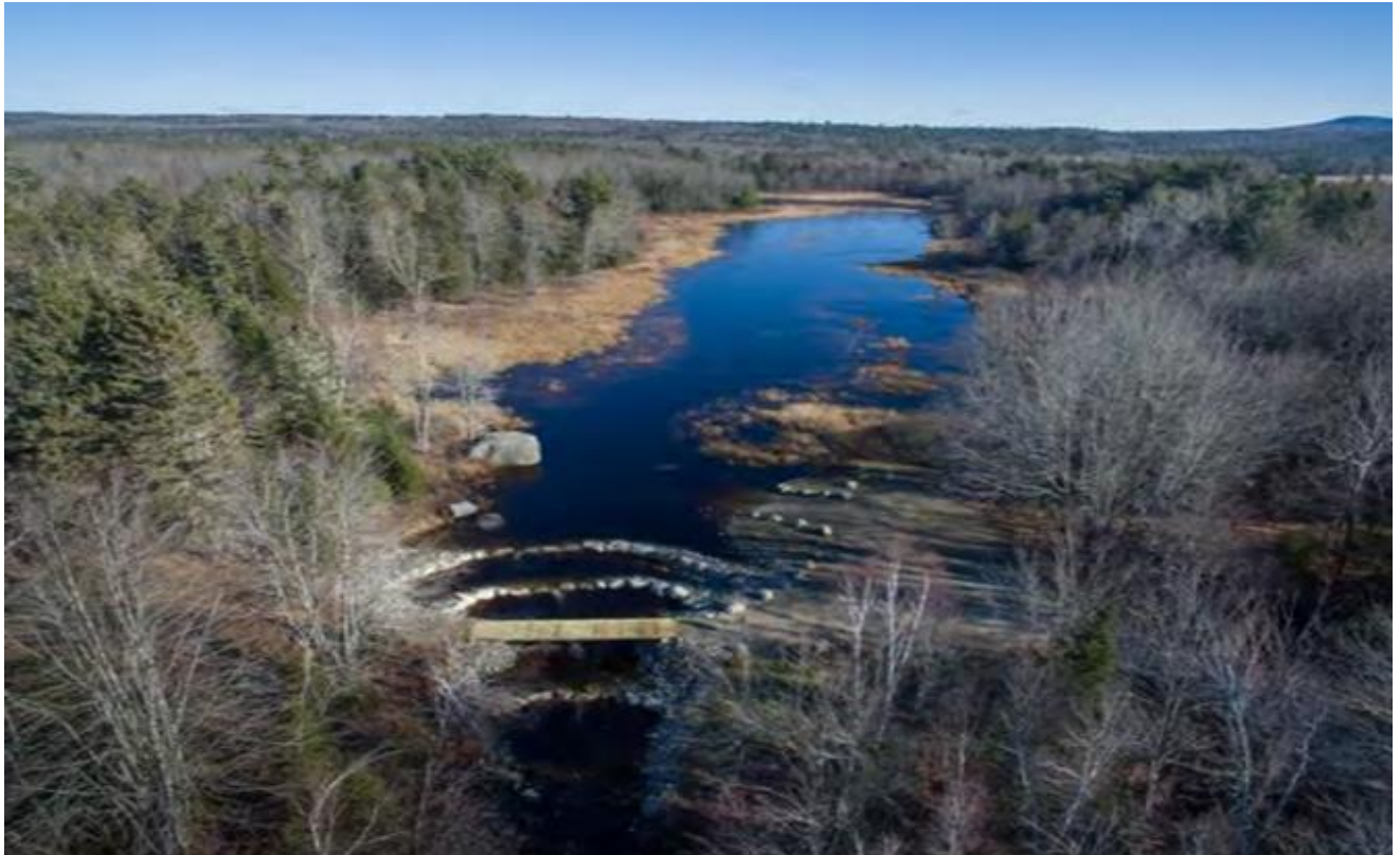
Nature-like fishway installed at Wights Pond
