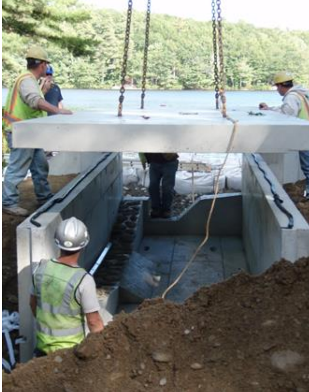
Installation of the new fish passage and removal of the existing outlet dam and fishway.
