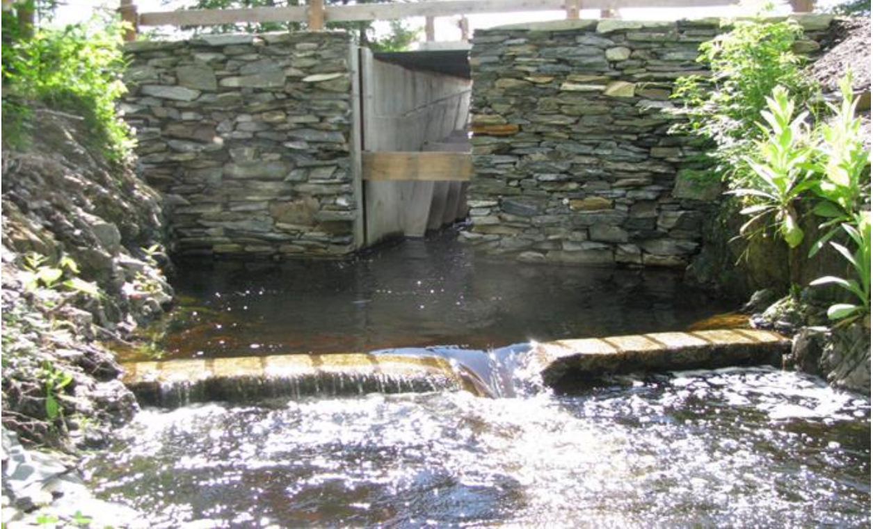
Newly constructed fishway through the outlet dam leading to Chemo Pond
