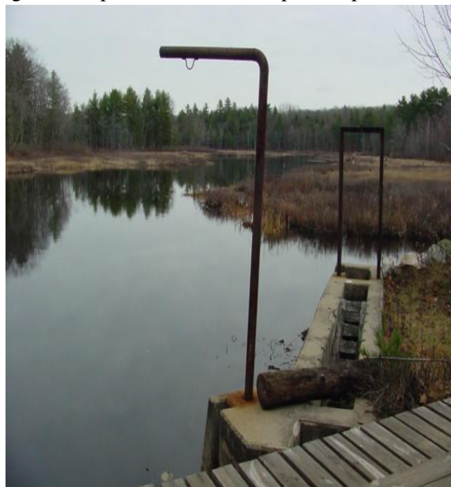
Outlet stream from Dyer-Long Pond, fishway leading into the pond and alewife trap at the pond outlet.
