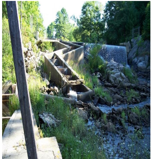
Historic picture of the Nequasset Mill and fish passage to spawning habitat and the trapping facility prior to 2014 rebuild.
