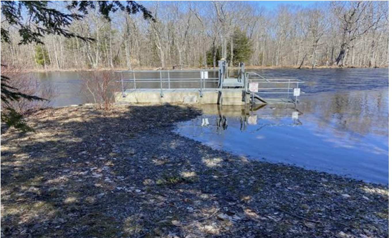
Newly installed fishway and overtopping of the dam during the river herring run.
