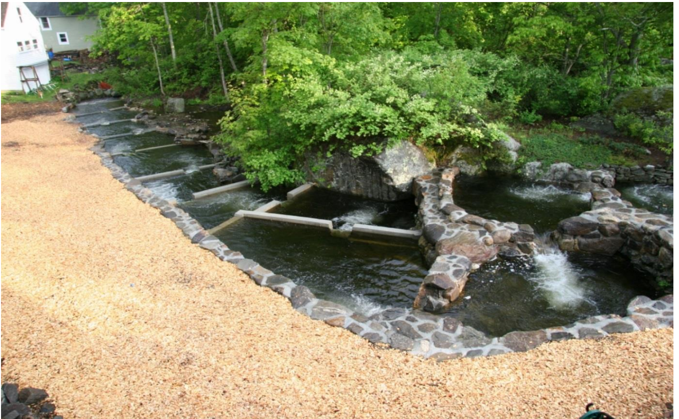
Upper section of the fishway after restoration.
